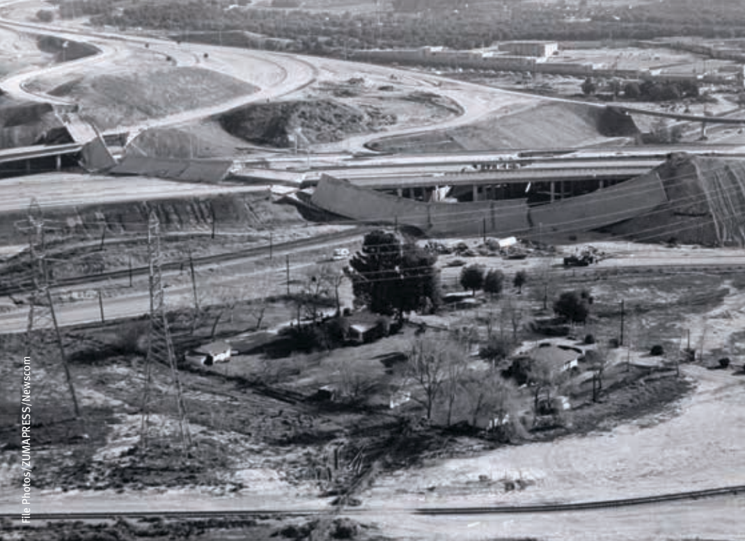
The Golden State Freeway at the Foothill overcrossing after the 1971 San Fernando earthquake (magnitude 6.6). Right: At least 15 people died in the Northridge Meadows Apartments during the Northridge earthquake in California (magnitude 6.7).
