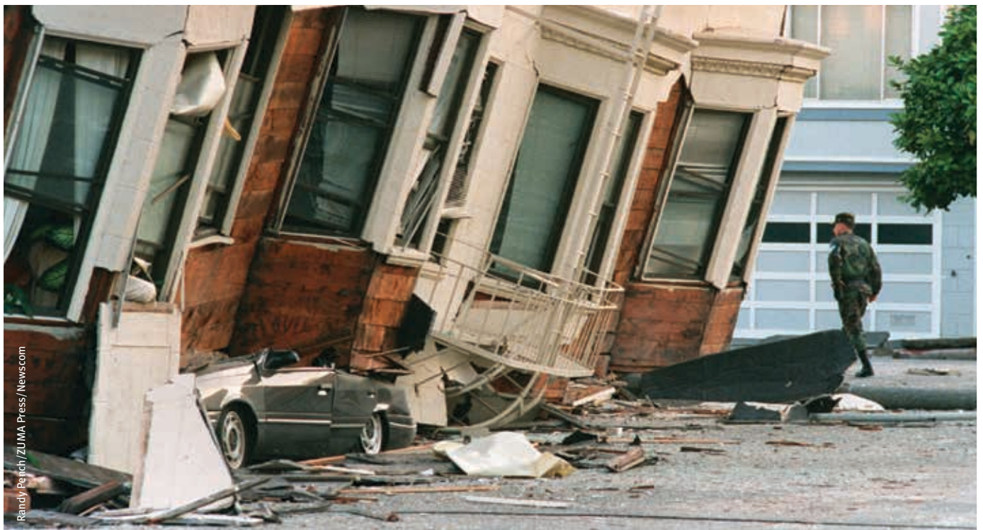
The crushed remains of a car sit under a collapsed Marina District apartment building, October 18, 1989, the day after the massive Loma Prieta earthquake struck Northern California.
