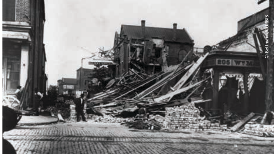
A magnitude 6.6 earthquake on Aug. 31, 1886, destroyed or damaged most buildings in the Charleston, S.C., area, including these homes on East Bay Street in Charleston.
